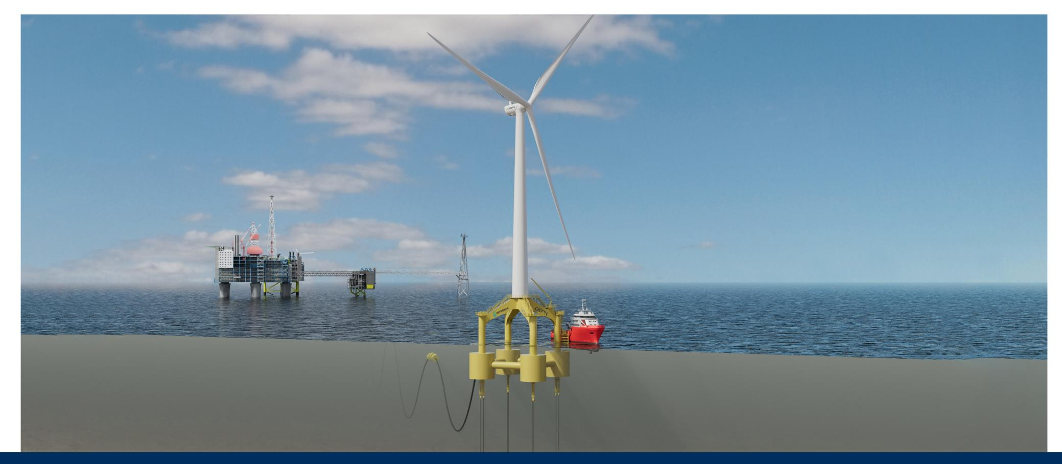
Development of a TLP-substructure. The modular topside is designed to be installed on a TLP-substructure. Due to different water depths and metocean conditions as well as different topside configurations, sizes and purposes, the TLP-substructure is designed scalable according to its required load bearing capacity.
